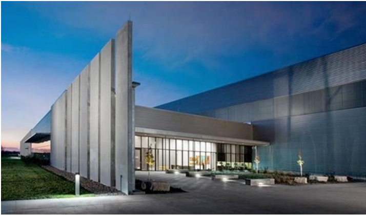
Facebook data center at Altoona, Iowa
